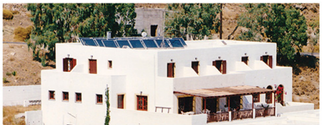
24 m 2 selective surface of copper collectors, Hotel in Amorgos, Greece
